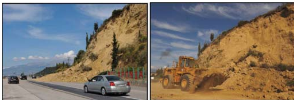
Figure 6. Landslides along the national road from Patras to Pyrgos near Vrachnaiika.
